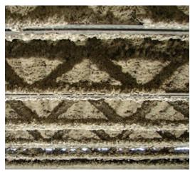
Figure C-4: Fireproofing added to structural steel
